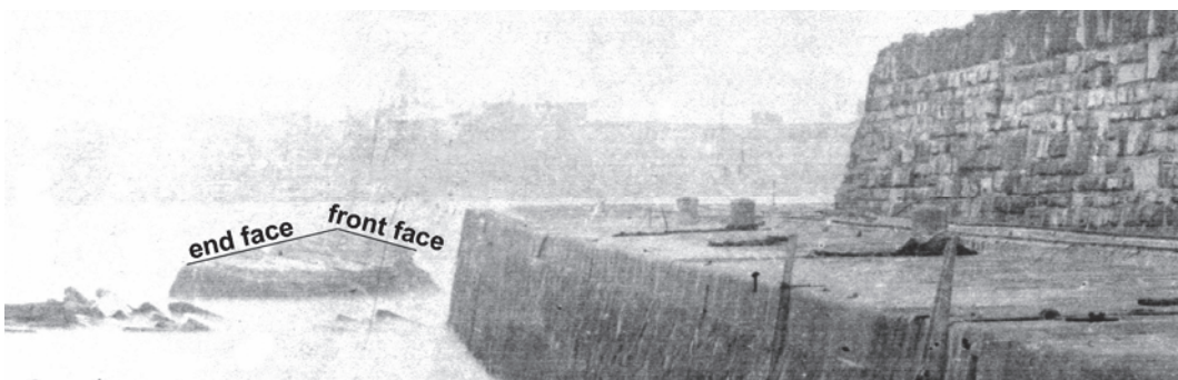
Figure 18. Part of detached end after December 1872 storm. ©The Wick Society 17
