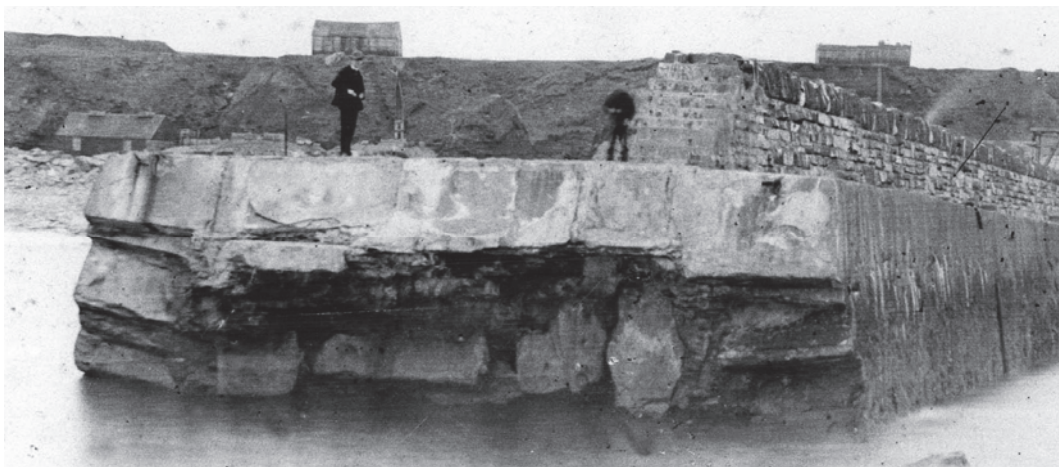
Figure 17. Stump end after December 1872 storm ©The Wick Society 17
